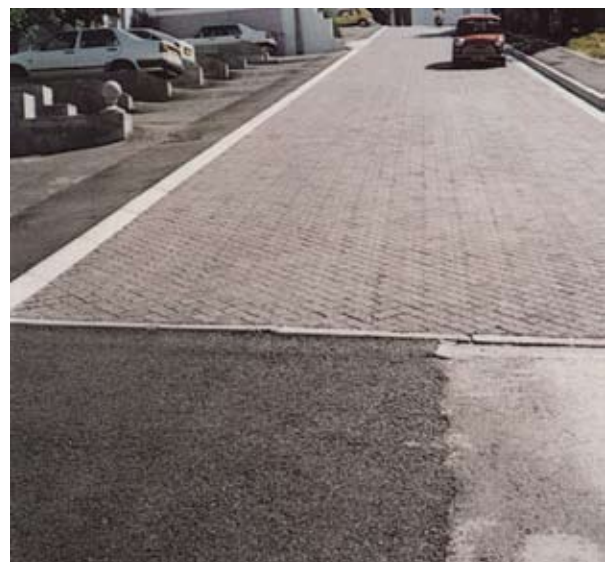
Photograph 9 – Upper Rhine Road - after rehabilitated
