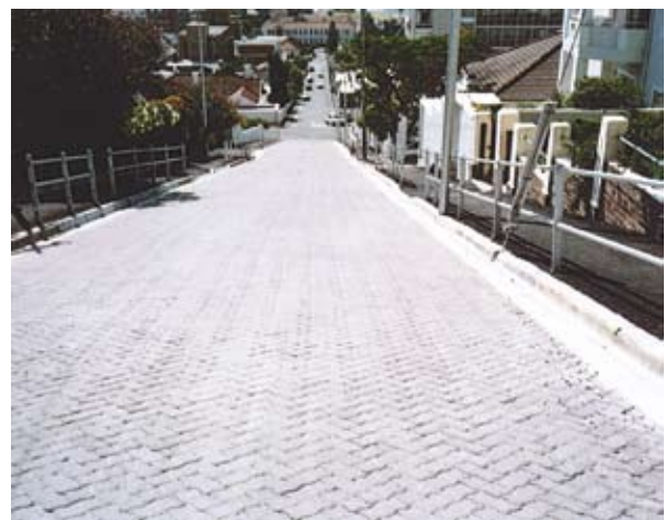
Photograph 2 – Boundary Road after rehabilitation
