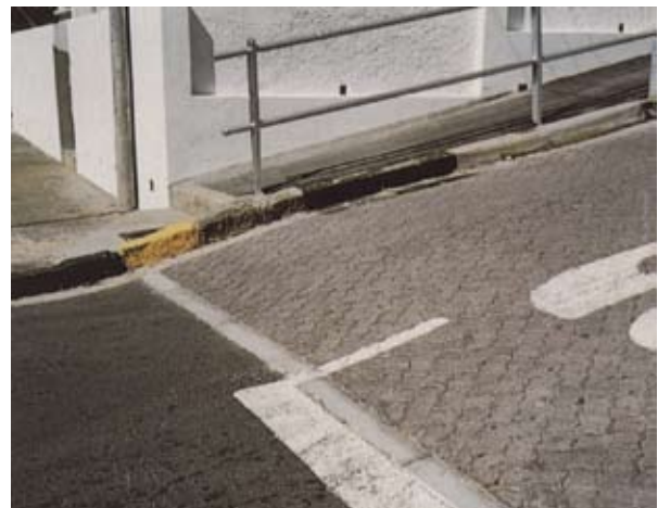
Photograph 3 – Anchor beam at bottom of Upper Rhine Road
