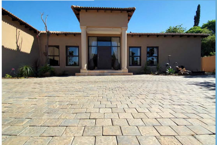
Residential premises, Somerset West
