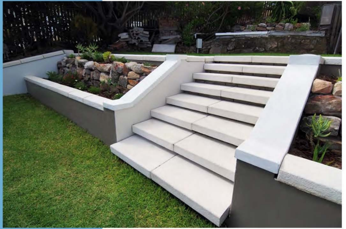
Residential premises, St James
