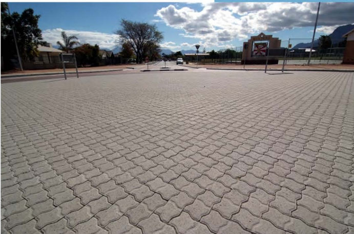
Mountain Mill Rd, Worcester
