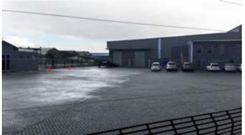
Standard interlockers on left and Permealock on right after rain.
